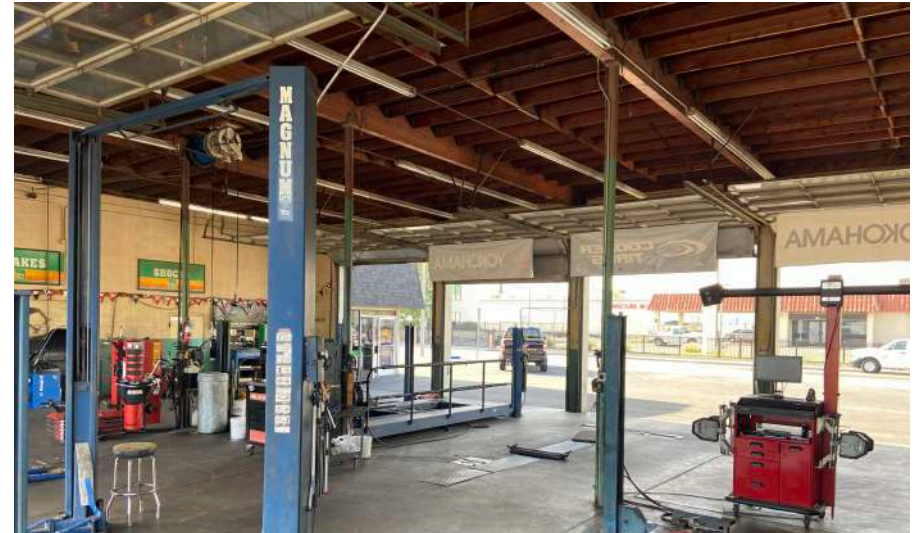
Open Air Service Bays
